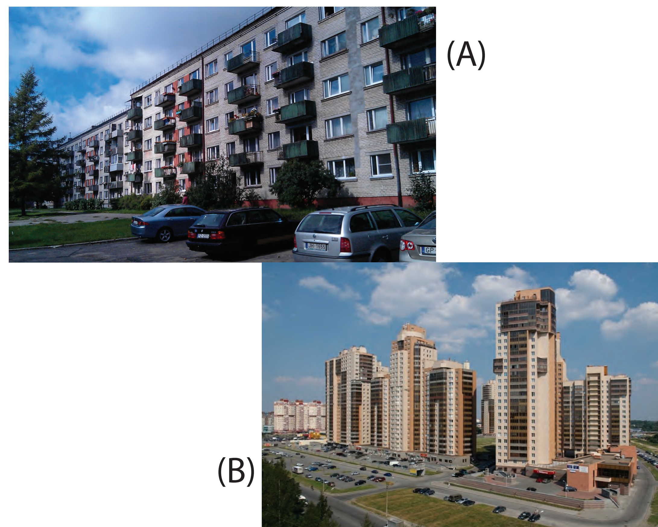
(A) This is a common Russian unit (or, in general, lingering Soviet era housing type) called the Khrushchyovka, named after Nikita Khrushchev, who began the massive urban housing initiative back in the 1960s, to house every Soviet. (B) This is an example of some of the newer housing options available to Russians that live near Saint-Petersburg. These homes are generally along the borders of the city, but they are just far enough to be outside the reach of the metro system.
